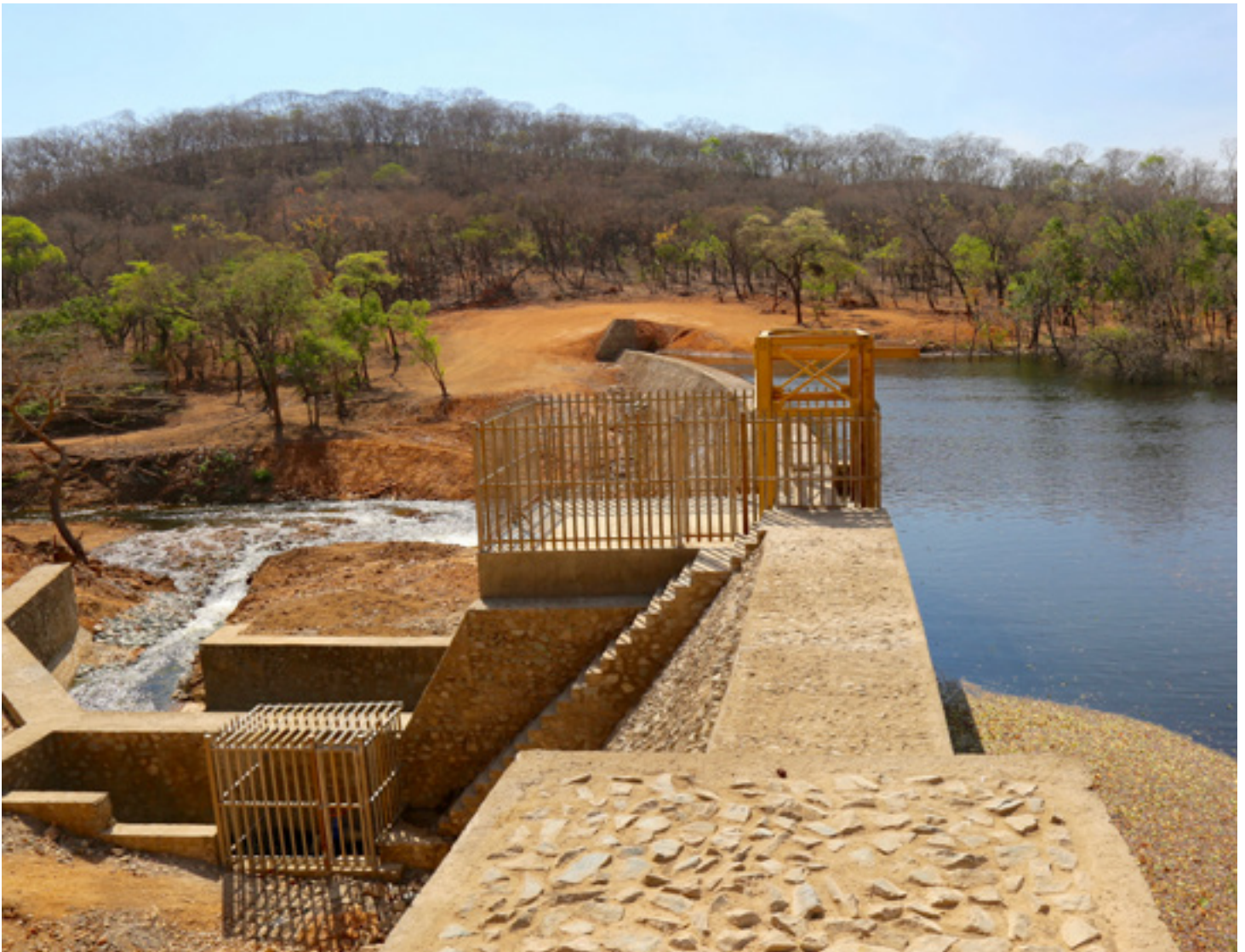
Luika River dam
