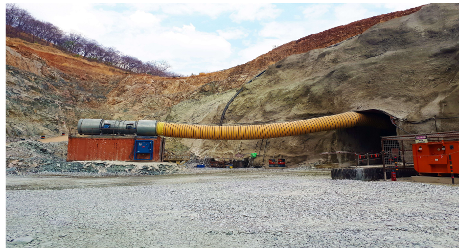
Ilunga underground portal (October 2018)
