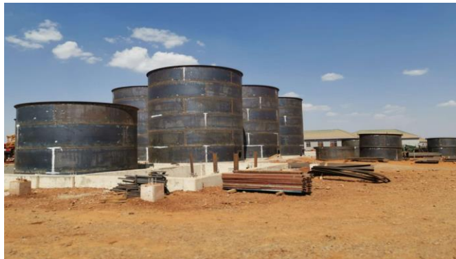
CIL Tanks Fabrication & Installation
